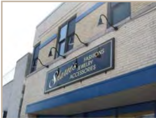
Generally, the appropriate zone for signage, including the brackets for projecting signs, is above the storefront windows and below the sills under the second-floor windows. This wooden sign uses carved gold leaf lettering on a black background. Four gooseneck lamps light the sign at night.
