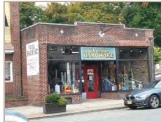
This carved and painted wooden sign uses gold leaf for lettering. This sign is well positioned over the door and between the transoms. This is an effective location for a quality sign.
