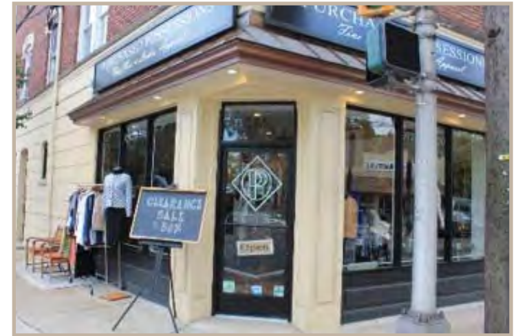
Retain original door locations, particularly on the main façade, such as this corner entrance shown above.
