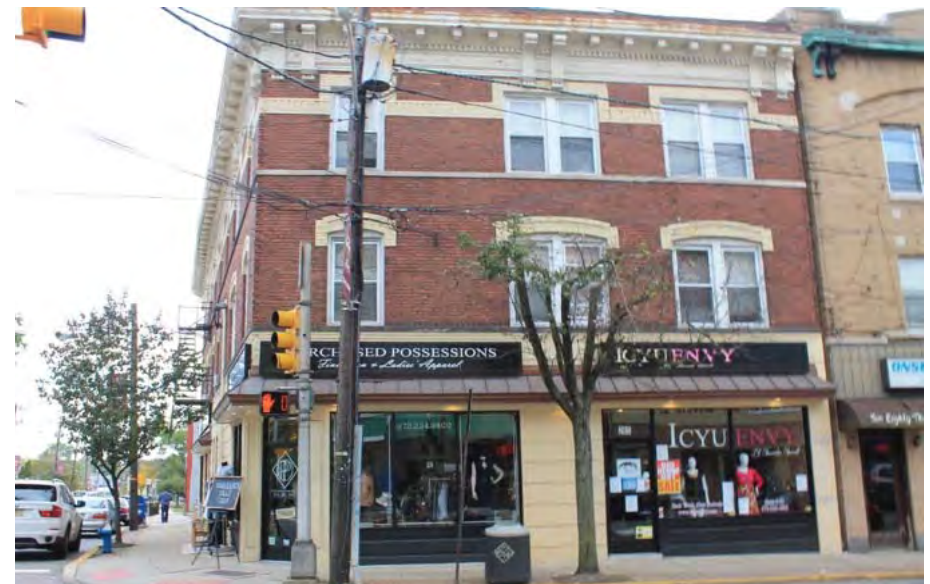
This property in Tory Corner was recently rehabilitated with two stores on the first floor and apartments above. The owners maintained and restored the cornice, cleaned and tuck-pointed the brick, and added new, modern but compatible storefronts for these thriving businesses.
