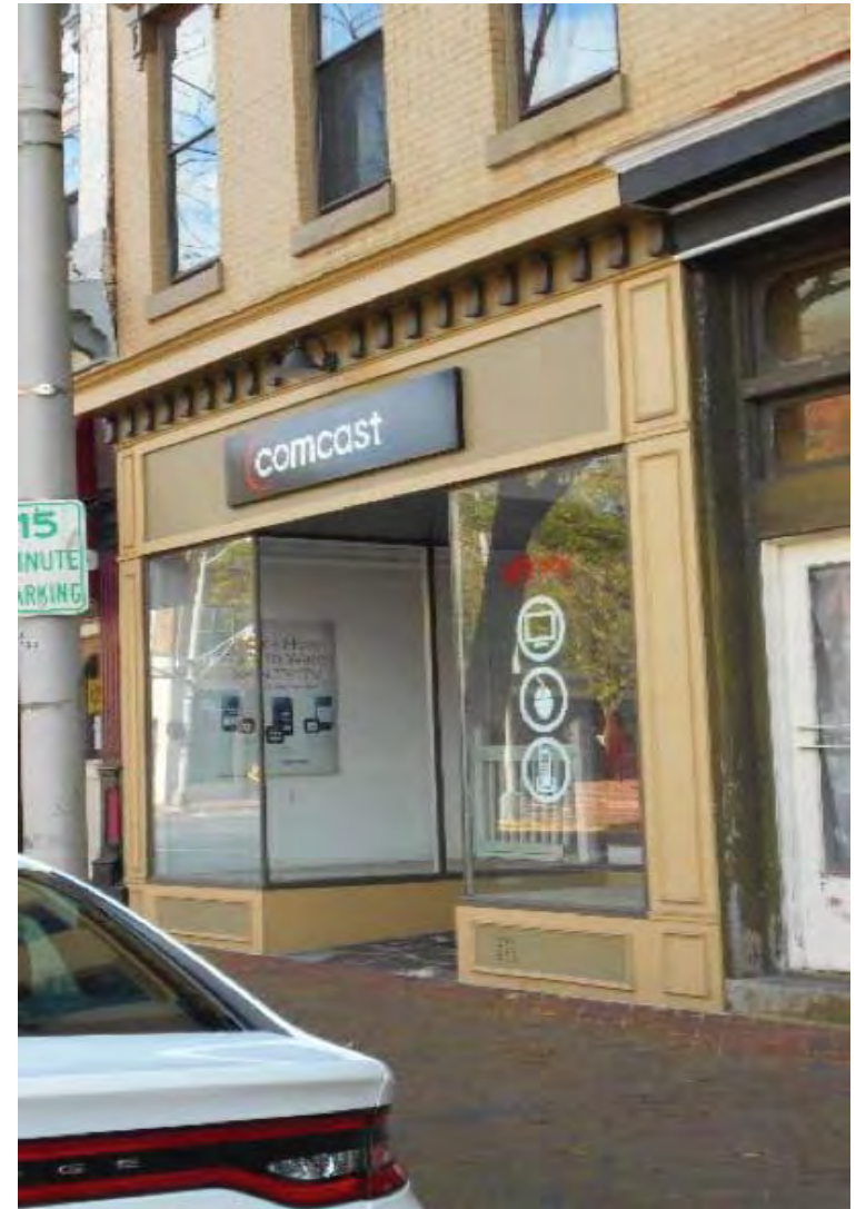
This storefront is neatly painted in colors to match the entire building. There is a high quality but simple metal sign using the logo of the company in the shop. There is one gooseneck light over the sign installed in the small bracketed cornice over the storefront. This storefront retains the original recessed entrance, wooden bulkheads, and large display windows, but the shop owner does not take advantage of the display space by merchandising the windows with their wares.
