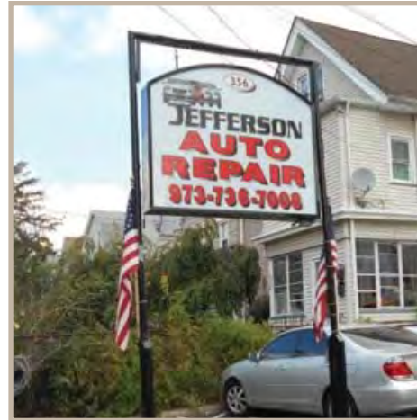
Freestanding signs should be supported by two wood, metal, or granite posts that, generally, are square in cross section.
