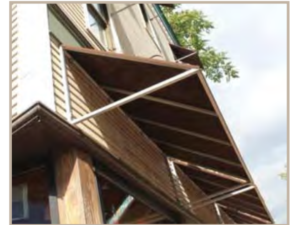
Use the traditional triangular awning shape, with either closed or open sides, for locations fronting the street. An awning with a loose valance along the bottom edge of the awning has a more traditional appearance than one that either has no valance or is fitted to rigid piping, but both are permitted.
