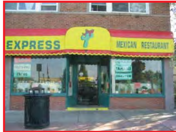
Bubble or rounded awnings on main facades, as these were not typical and tend to hide important architectural features, are not recommended
