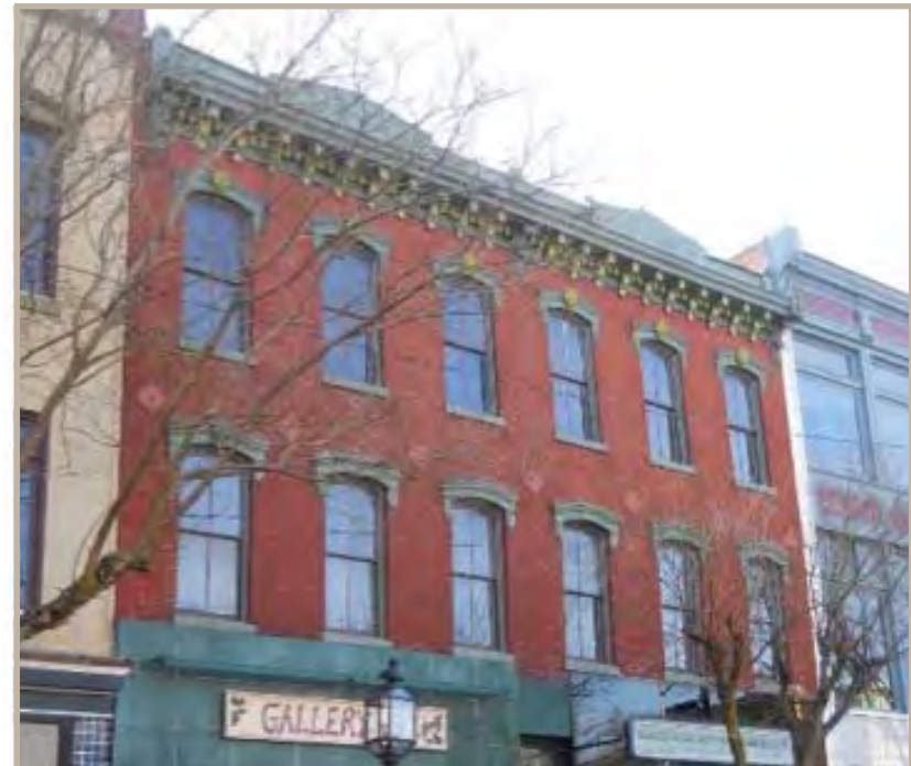
Retain any decorative features around upper story windows. If deteriorated, make repairs to decorative window hood molds (wood, brick, or metal features over the windows) shown here.
