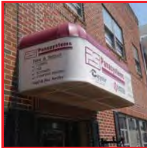
Back lit or internally lit awnings with plastic grates to cover bulbs are not recommended.
