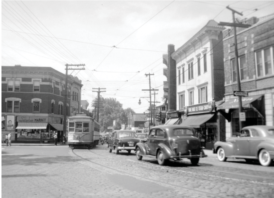
This original storefront still retains the wooden bulkhead, recessed entrance, original display windows, and an older but still effective wooden painted sign correctly positioned in the sign band at the top of the storefront. The merchant displays current merchandise and signage to promote their business in their display windows.
