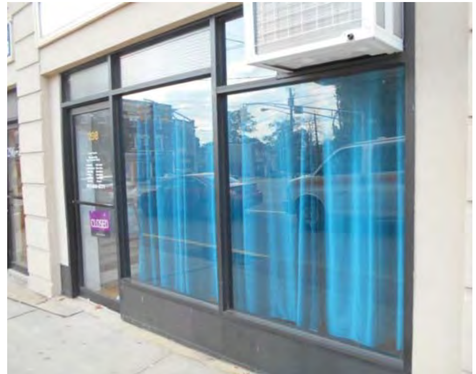
The property owner here in Tory Corner has installed a simple and clean compatible modern storefront onto an older building. The brown aluminum storefront maintains the street wall, retains the transom area above the display windows, and has a metal bulk head that supports the window glass. There is a small painted sign on the door glass. The shop owner uses blue drapes to regulate the sun coming into the windows and provide privacy for their clients.
