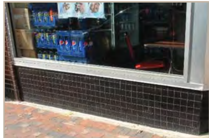
Bulkheads can be made of wood panels, tile (seen here), polished stone, glass, or aluminum-clad plywood panels.
