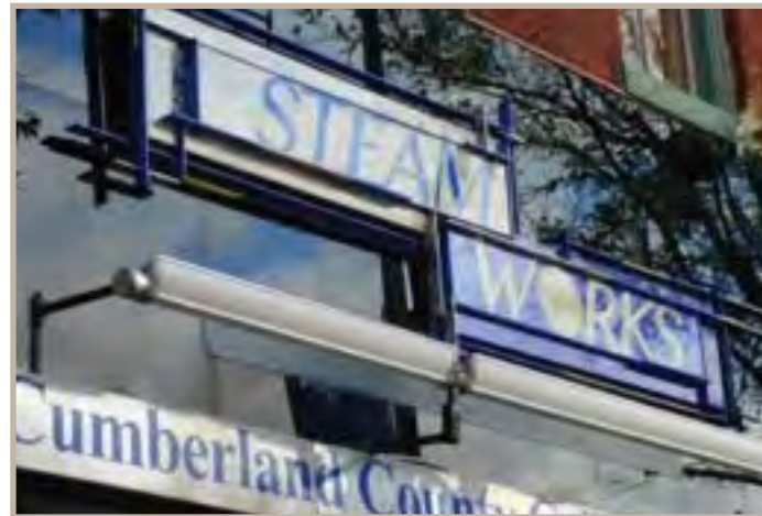
Signs may be externally illuminated by one or more shielded, stationery bulb projecting onto the sign. Here, the handsome sign for Steam Works is illuminated from below using long lighting fixtures.
