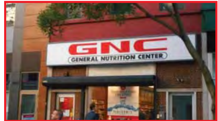
Internally lit signs, like this one here, are prohibited on the exterior of buildings in the downtown. The plastic feel of internally illuminated signs is inappropriate in our historic downtown.
