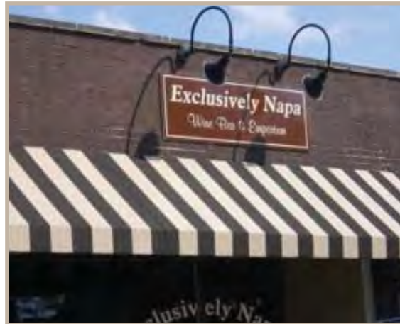
Traditionally, awnings were either solid colors or striped. In choosing a pattern, be guided by the building itself. A striped or bold awning may enhance a plain building, while a more decorative building may require a solid color awning in a subtle shade. This brown and white awning adds interest to an otherwise plain brown painted brick façade.
