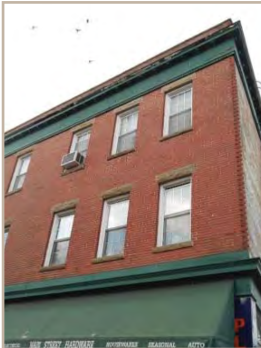
Retain any upper story windows as windows.
