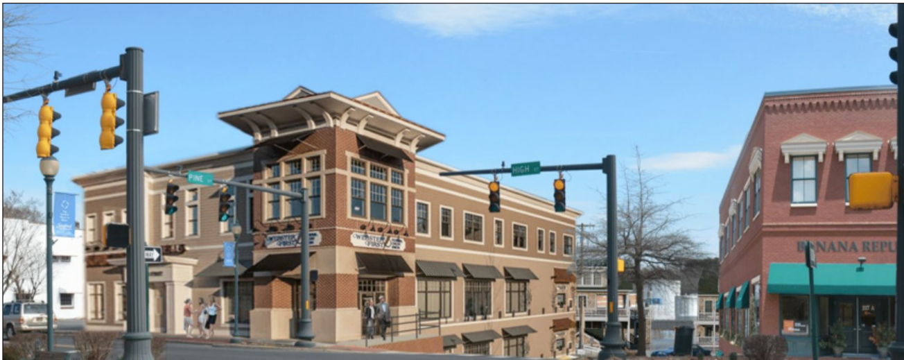
This rendering of a proposed redesign of two buildings on High Street was included in the 2016 Seaford Community Vision Plan. This rendering shows how high quality, compatible new construction can add to the street life of downtown Seaford. Both of these buildings retain the existing street wall, are made of building materials consistent with existing downtown structures, maintain the solid (wall) to void (window) relationships, and retain the same scale, height, and massing as existing buildings. These two buildings would be highly successful new buildings that retain the historic character of downtown Seaford.
