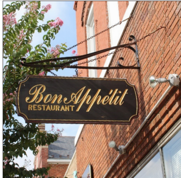
The bracket for this perpendicular carved wooden sign is located in the correct location for a historic building, which is in the sign band, situated above the storefront display window and below the second-floor windows.
