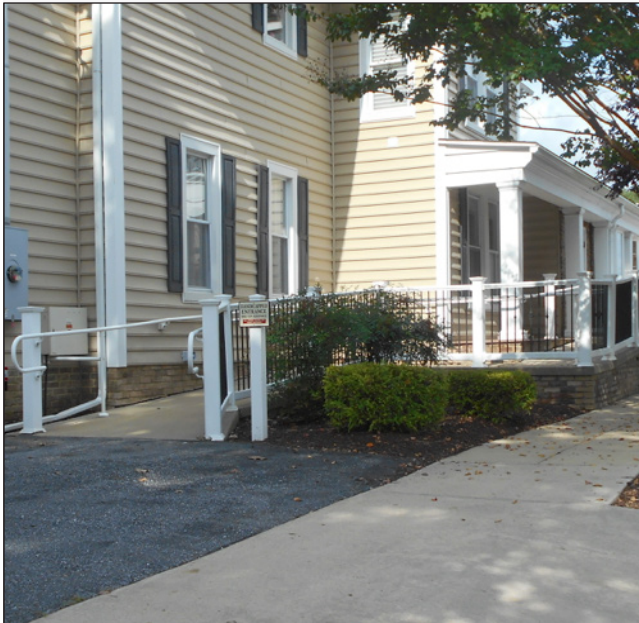
Implement improvements according to the Americans with Disability Act (ADA) standards for handicapped accessibility as they have done at the Prociano, Wells and Woodland Law Firm located at 225 High Street.
