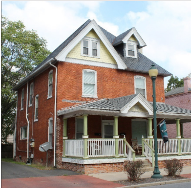
128 High Street is constructed mostly of brick, but the wooden porch columns and balusters, along with the fish scale shingles in the gable are all painted attractive colors that complement the masonry structure.
