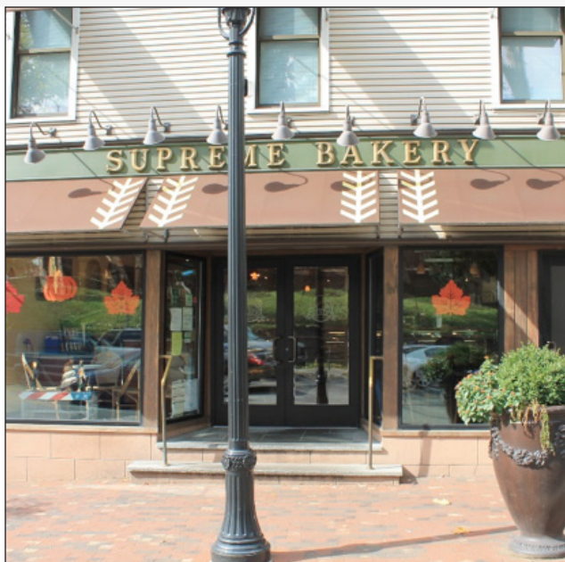
Keep traditional storefronts as transparent as possible and retain the existing glass storefront windows whenever possible. If window glazing is being replaced, make sure that the new windows are transparent and not tinted. This bakery in West Orange NJ uses large open display windows to show the bakery cases filled with cakes and pies within.
