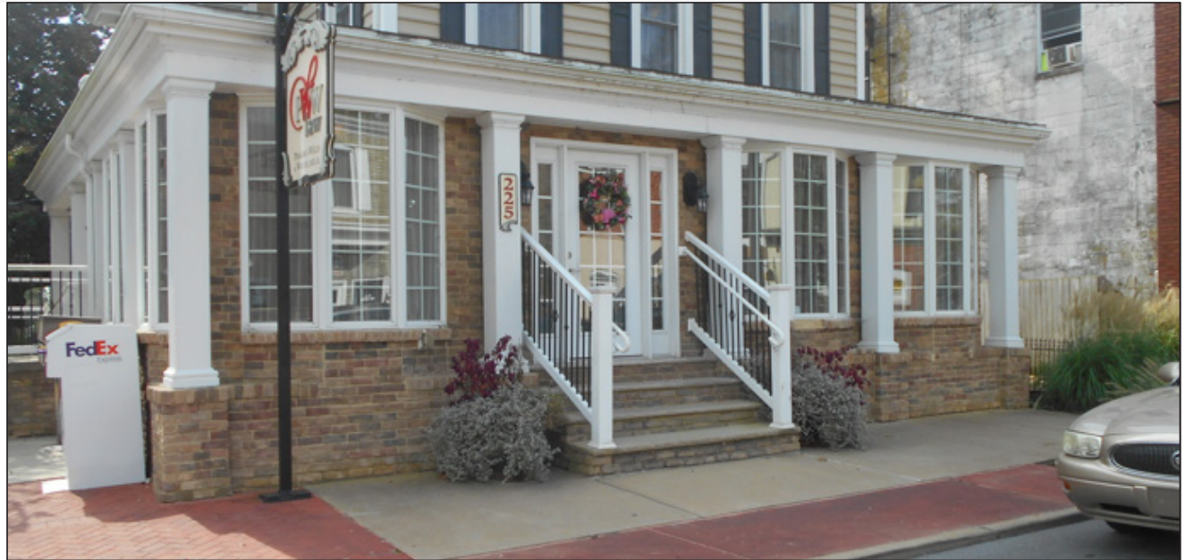
225 High Street is a professional office that has well-placed and maintained flowering planters, as well as clean sidewalks. Upkeep, such as this, makes a great first impression for shoppers, diners, and visitors to downtown Seaford. Seaford Spade and Trowel offers bedding plants and planting of street containers twice a year for a fee for interested property owners, see an example of their work here. Property owners are responsible for watering and general maintenance for planters and street containers.
