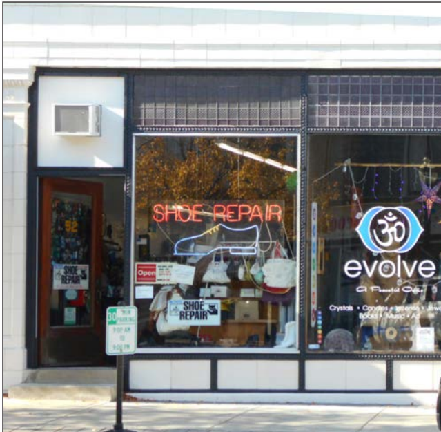
This traditional storefront in Milford DE retains its original wood glazed door, the Luxfer glass transoms above the display windows and wooden bulkheads below the display windows.
