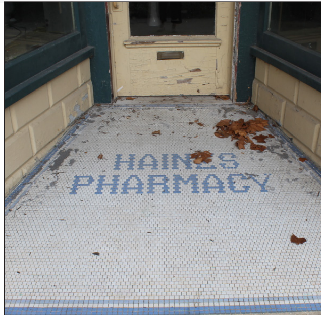
Repair and retain any existing tile work or decorative tile or terrazzo flooring on the exterior entrance flooring, like this one for the former Haines Pharmacy once located on 324 High Street.
