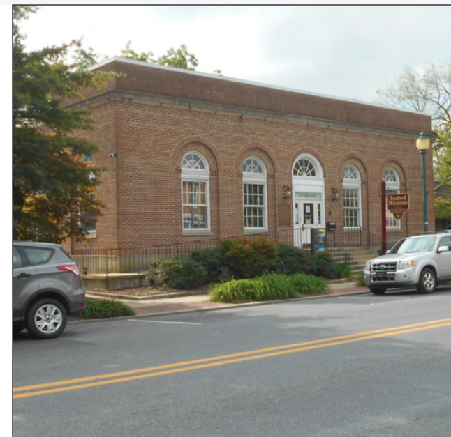
The best choice for replacing a historic wood window is to use a new wood window. The wood should be painted to protect it from the elements. The Seaford Museum, located in the former Post Office at 203 High Street, retains all of its original wood windows.
