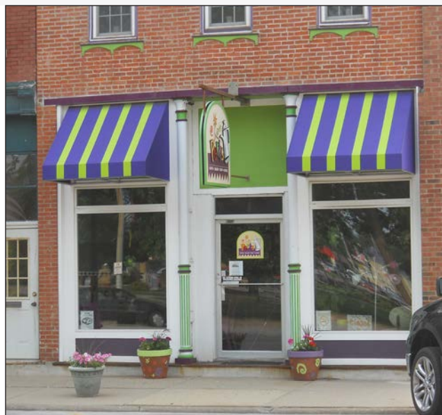
Let the design of the building determine the number of awnings to be used. A single storefront (without structural divisions) will usually require a single awning. A building with separate display windows and doors may need separate awnings that correspond to those divisions. This building in Philadelphia PA uses multiple striped canvas awnings, in vivid colors, to differentiate their handsome storefront.
