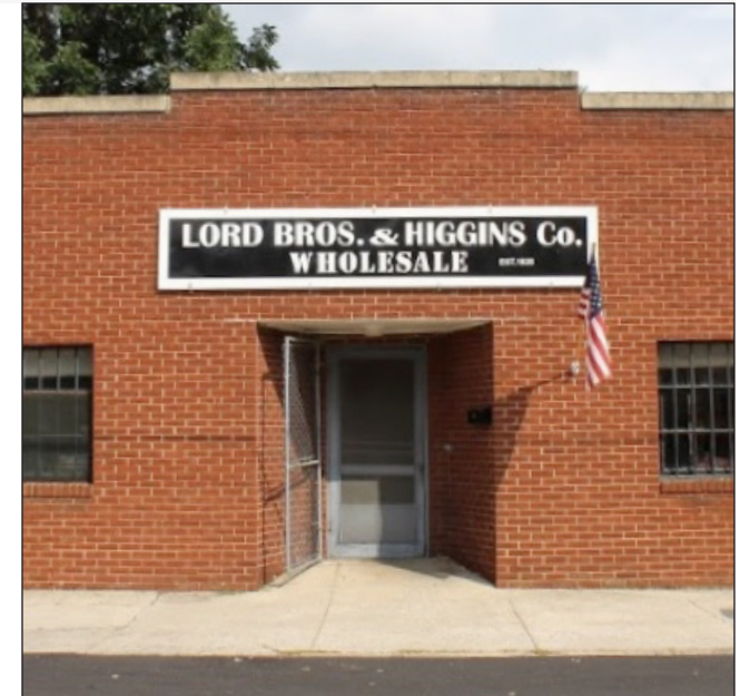
Commercial buildings typically have a long, thin (usually less than three feet wide) area above the storefront where a sign would traditionally be located. This area is often called the sign band and is an appropriate location today for signage, like the example here for 125 North Conwell Street for Lord Bros. & Higgins Co. in Seaford.
