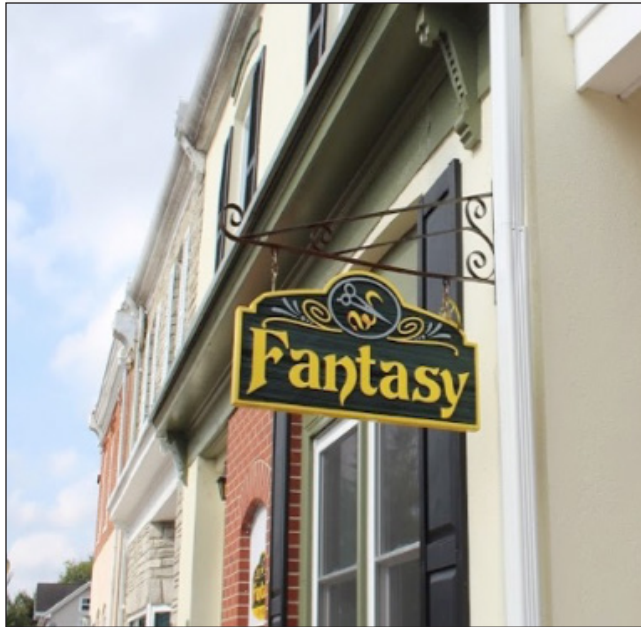
This small, painted wood projecting sign for the Fantasy Hair Salon at 224 High Street is appropriate for a historic building in Seaford.
