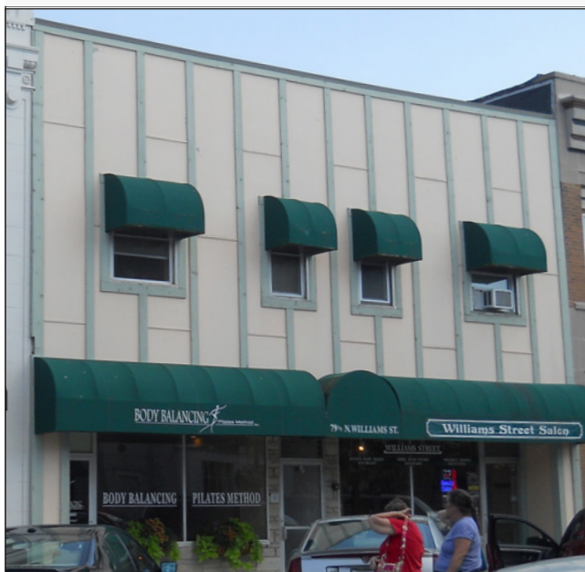
Covering any part of the building façade with stucco or other siding is not recommended as seen here in Crystal Lake IL.
