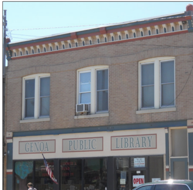
All the upper story windows in this Genoa Illinois building are made of wood and fit the shape of the window openings.
