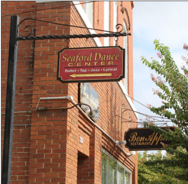
These two wooden signs at 312 High Street are hung in the sign band, are placed perpendicular to the façade, and are carved and nicely painted. They both stand out on the street. One is a freestanding sign hung from a simple metal pole, the other is a projecting sign hung on a metal bracket mounted on the brick façade on High Street in Seaford.
