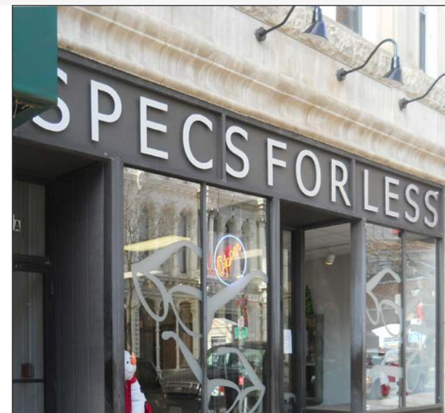
If an original storefront is missing altogether and an incompatible modern store front exists in its place, rehabilitation can be accomplished by building a new storefront, like the one seen here in Wilmington DE. Here the new compatible storefront fits within the original limestone frame, and uses simple modern brown aluminum for the bulkheads, sign band and frames for the display windows.
