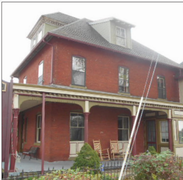
All of the original windows have been retained on this historic home at 413 High Street.
