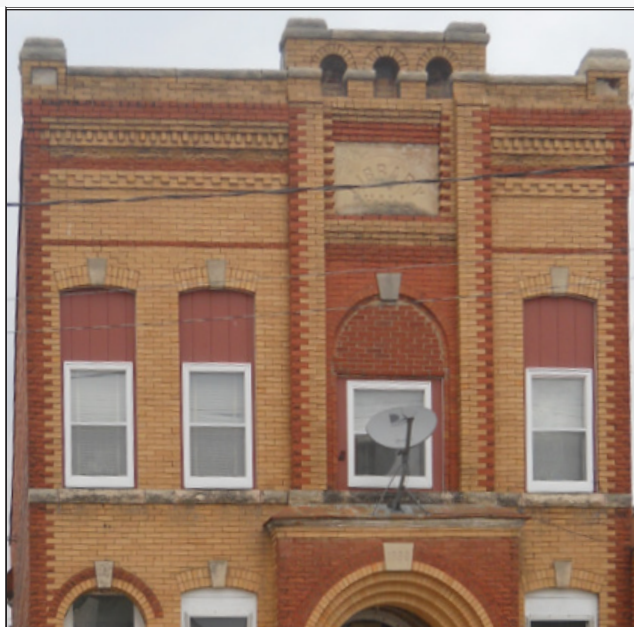
Reducing the size of the windows by replacing them with smaller sized windows in this otherwise handsome and intact historic building in Cambridge IL, is not recommended
