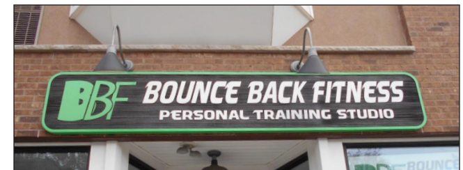
A small, well-crafted sign from Metuchen New Jersey, fits within the traditional sign band on this two-story building and has gooseneck lamps that illuminate the sign at night.
