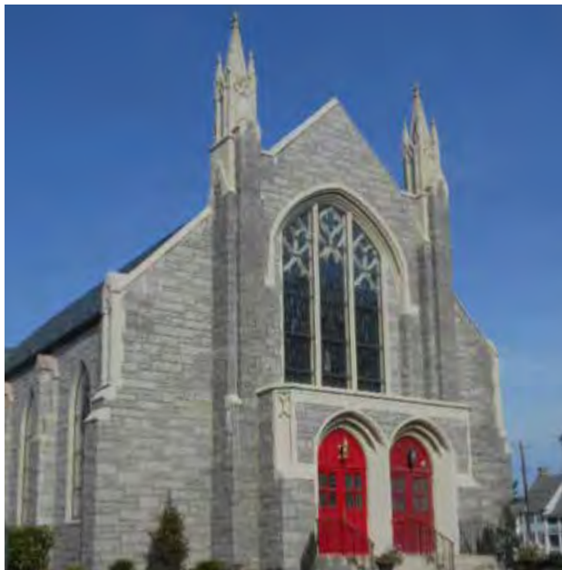
20 North Church Street. Avenue United Methodist Church is constructed in the Gothic Revival style. Limestone is used to highlight the edges of the gable, the tracery of the large stained-glass windows over the entrance, the entrance doors, and the spires on the towers on this gray stone building.
