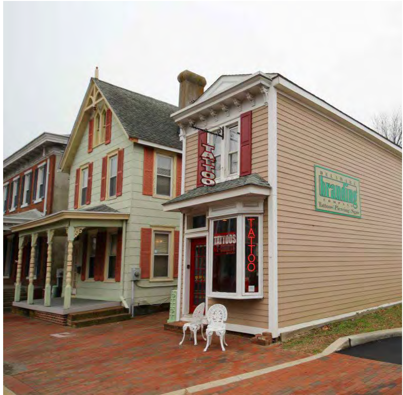
This small and charming building has been well maintained and now houses a tattoo shop.
