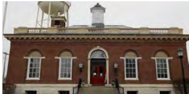
Left: 121 South Walnut Street, now the Milford Museum, is a fine brick building in the Colonial Revival style. This building has a limestone base and cornice, and uses limestone trim around the central door, around the tall six over six windows, and for the baluster and paneled parapet wall at the top of the roof.
