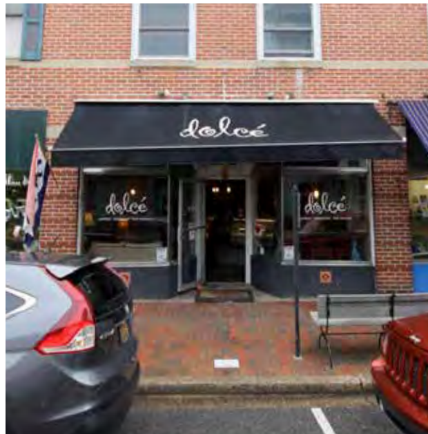
This Milford storefront retains the historic metal window frames, its inset entry vestibule and transom windows. The retractable black canvas awning permits the shop owner to regulate the amount of sun coming into the building during the day.
