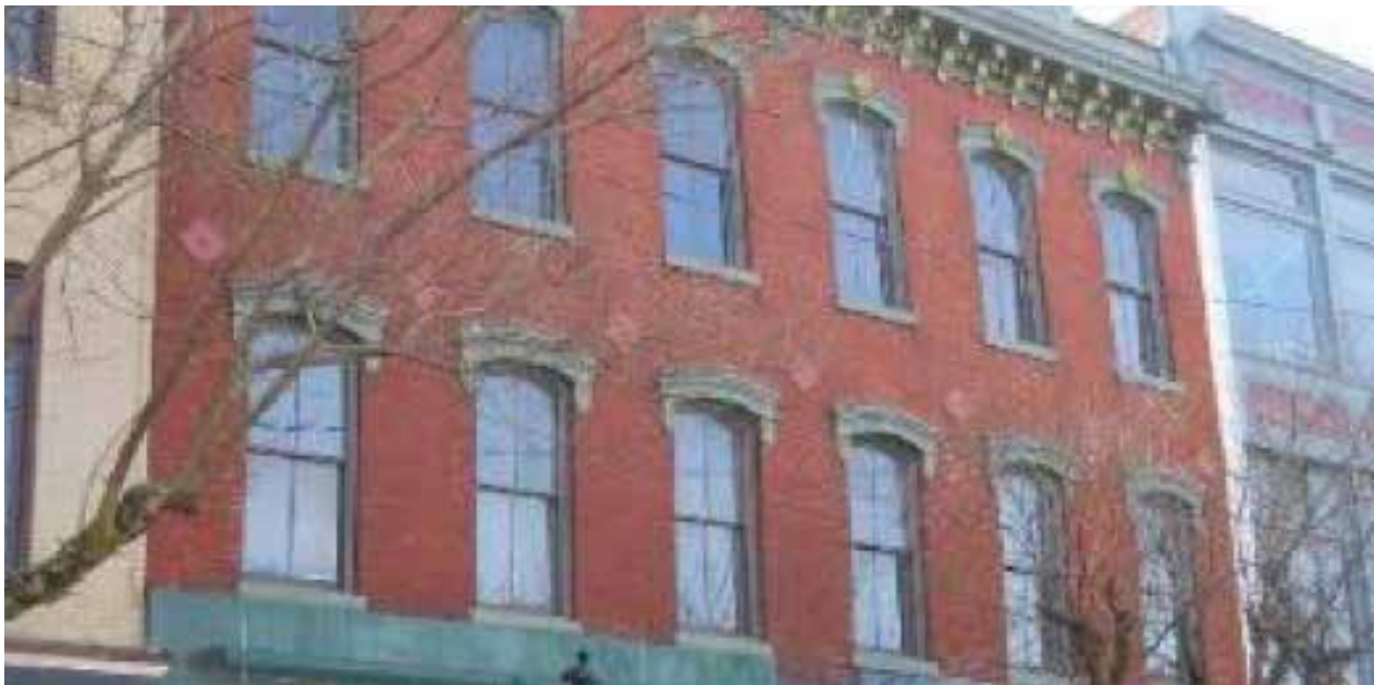
The two over two light replacement wood upper story windows for this building in Bridgeton NJ fill the entire window opening.
