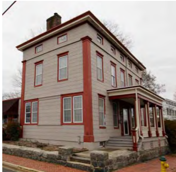
7 NW 2nd Street, Crown Upholstery, is a Greek Revival building made of wood. It has a series of attic story windows in the frieze, which are often seen in Greek Revival residential buildings. The tall pilaster corner boards are highlighted with rust colored paint on this building.
