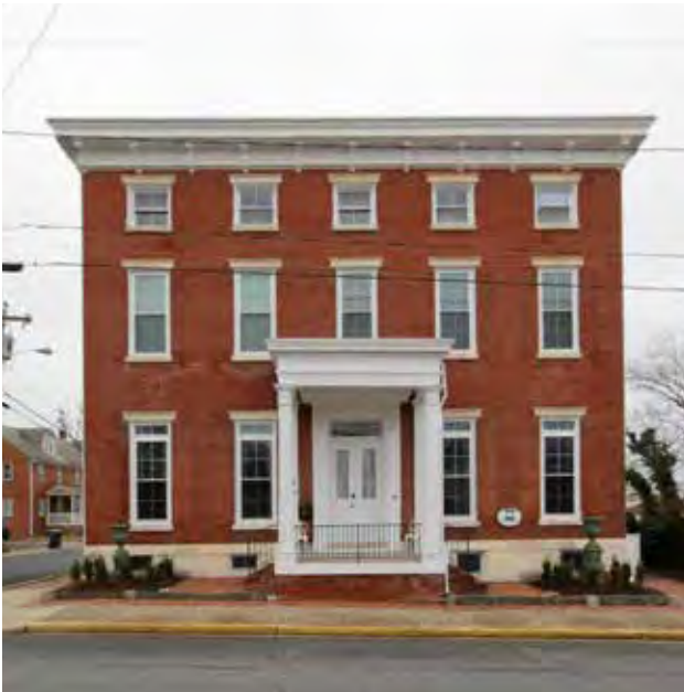
119 North Walnut Street, The Bank House Bed and Breakfast. This high style Greek Revival building has a porch with its original wood Corinthian Order column capitals, and a paneled double door with glass and a transom above.
