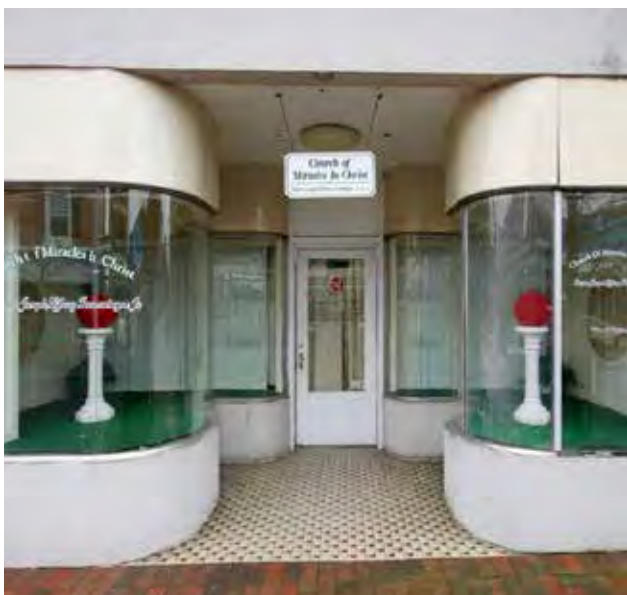
19 South Walnut Street is an excellent example of the Art Moderne style in Milford. The handsome curved storefront uses glass and beige Carrara Glass above to create a display space for this retailer. The black and beige tile pattern in the entryway reinforces the color of the Carrara glass.
