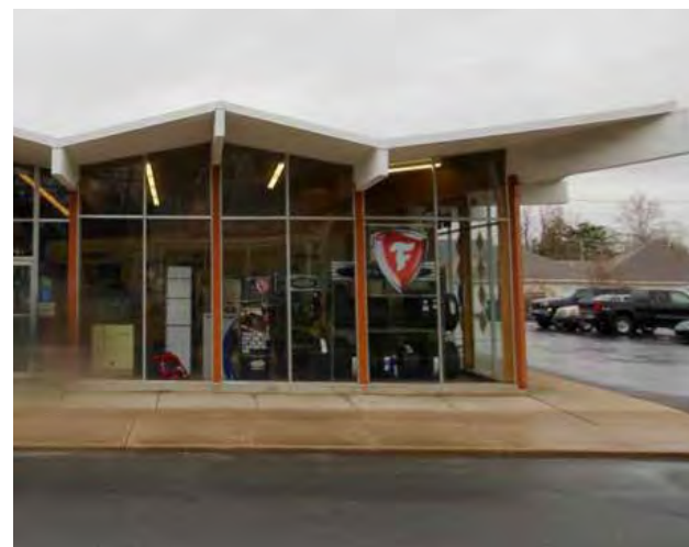
103 Causey Avenue, a Firestone Tire Dealer, is an excellent example of Mid Century Modern style architecture. The wide, zig zag shaped white cement roof sits on slim piers that permit the roof to cantilever out over the sidewalk to create a covered pedestrian passageway. Large floor to ceiling glass panels with aluminum frames fit between the piers to provide light into the showroom. This building is in a remarkable state of preservation.
