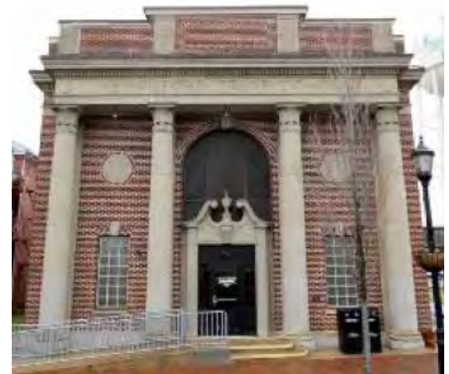
This Colonial Revival style brick and limestone former bank building now used as the Milford Customer Service Department at 119 Walnut Street. The original windows have been changed to glass block on the front façade.
