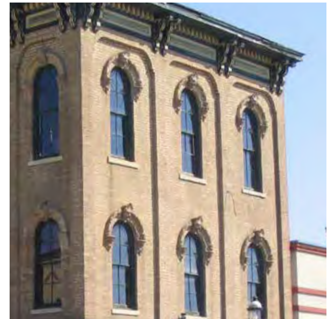
All the upper story windows in this Wilmington DE building are made of wood and fit the shape of the window openings.
