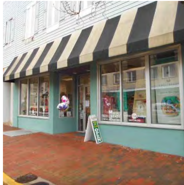
This striped canvas awning stretches over the entire façade and unifies the storefront.
