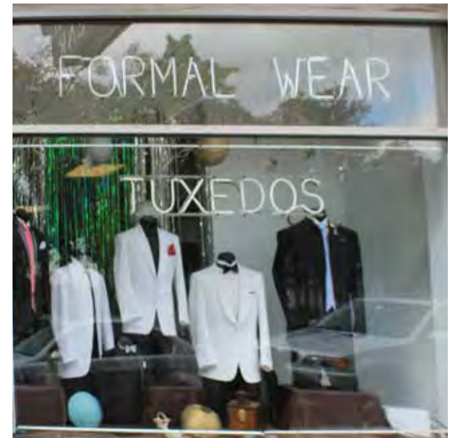
The shop owner of this modern metal storefront uses simple mannequins to showcase the formal wear sold and rented from this shop. Note the neon lettering positioned inside the window display glass.
