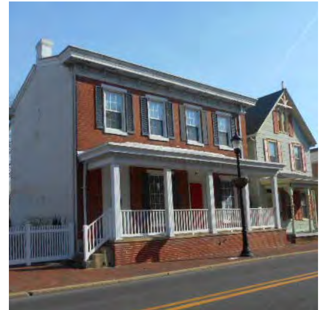
This small vernacular Greek Revival building is made of brick and has simple, square shaped, paneled pilasters that hold up the porch roof.
