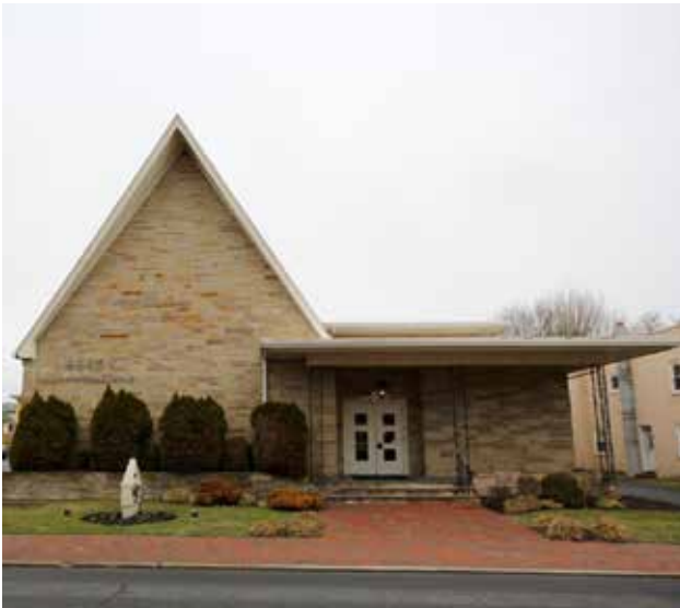
This Midcentury Modern style funeral home continues its original use and is well maintained.
