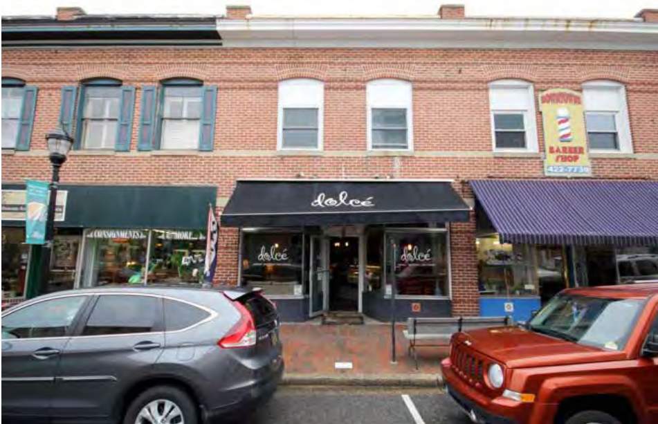
36 North Walnut Street is a vernacular style example of the Italianate style found in Milford. The simple metal cornice, limestone string course that links the window sills, and the segmental arched brick lintels on the second-floor windows are the only distinctive architectural features for this simple, vernacular building.
