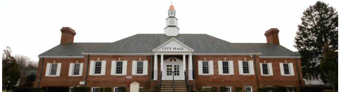
Above: 201 South Walnut Street. City Hall was completed in 1959, and is a very late example of the Colonial Revival style. The central entranceway is up a flight of stairs and is composed of paired wooden columns with Doric order capitals that hold up a simple gable. The building sits on a high brick basement and has a pair of large brick chimneys at either end and a central clock tower.
