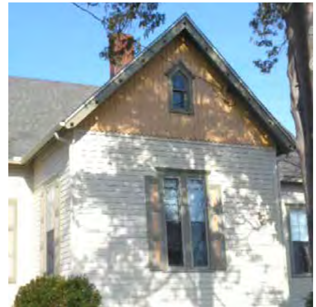
18 N. Church Street. The Milford Woman's Club is a vernacular example of the Gothic Revival style. The upper part of the gable is made of board and batten finish siding, and the vergeboard has simple cut-out decorative features. There is one pointed arch window at top of the gable.
