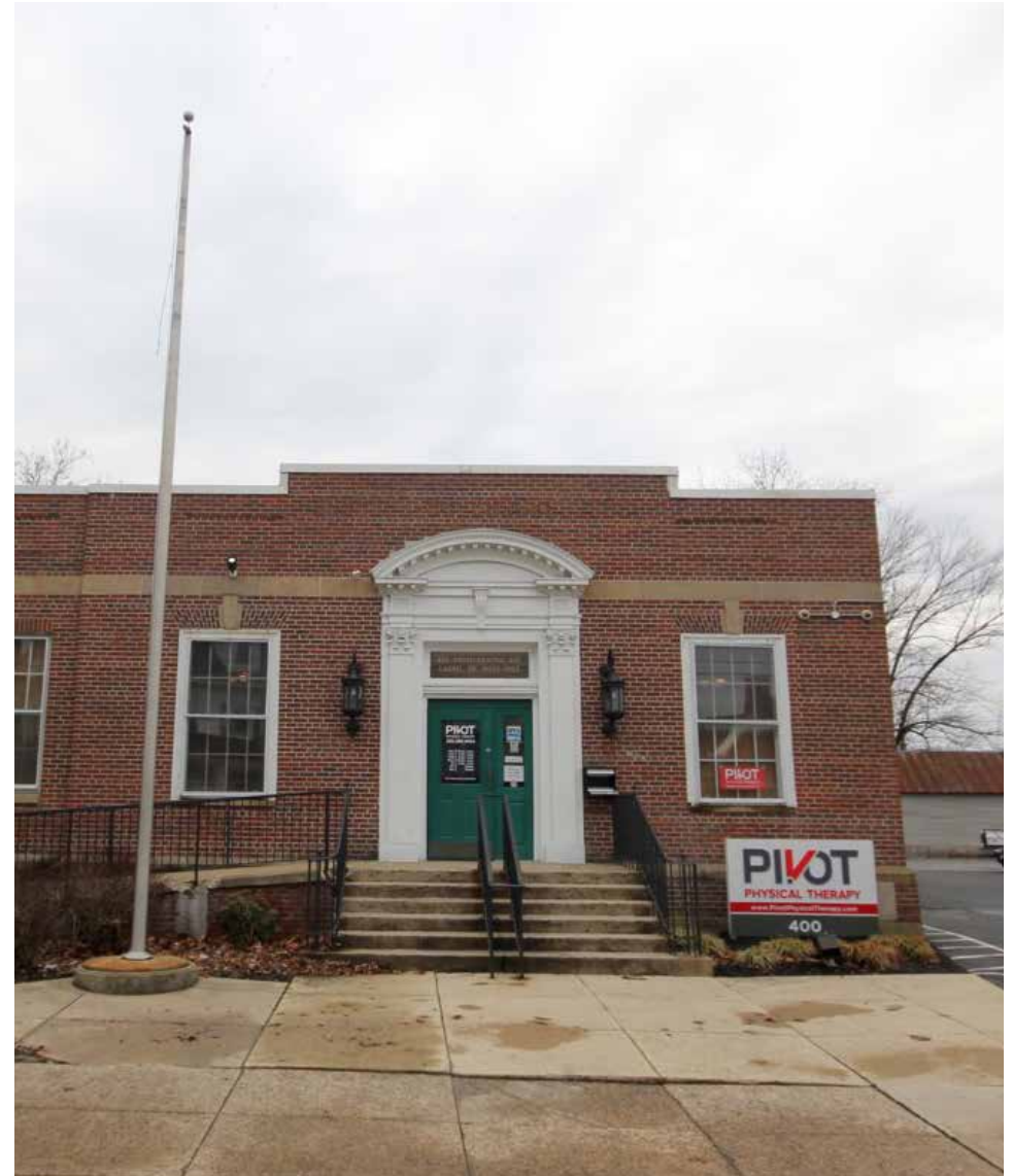
The former post office, now used by Pivot Physical Therapy, at 400 South Central Avenue in the Classical Revival style retains all its historic character and is well maintained today.
