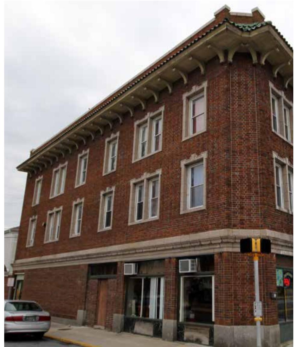
This mixed use commercial and residential use building at 124-126 East Market Street retains all the wooden upper story, one over one wooden windows.
