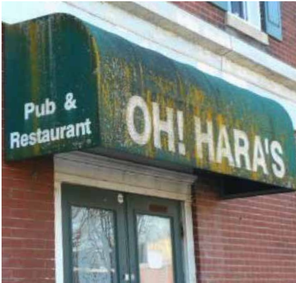
Maintain awnings in good condition, wash and repair them as needed. This awning needs to be washed or replaced.
