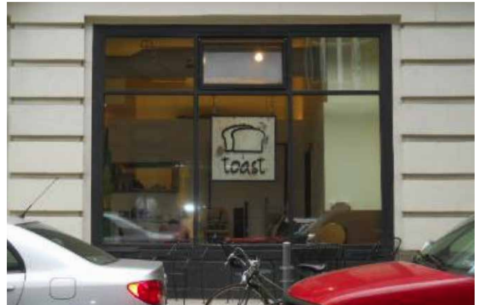
This storefront replacement window in Philadelphia uses a large amount of glass and a simple, straightforward design that blends with the building in terms of form, style, and material.
