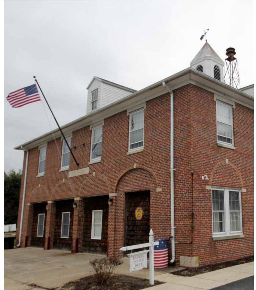
Town Hall, at 201 Mechanic Street, is a former firehouse that has been adapted for use as the municipal building. The Classical Revival style building retains its historic character and has been well maintained over the years.
