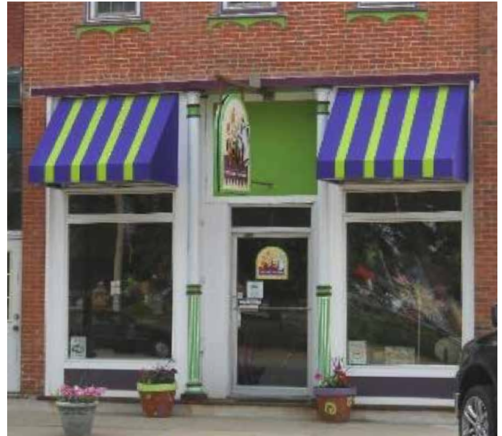
Let the design of the building determine the number of awnings to be used. A building with separate windows and doors may need separate awnings that correspond to those divisions, like this Philadelphia shop with two bold colored striped awnings.
