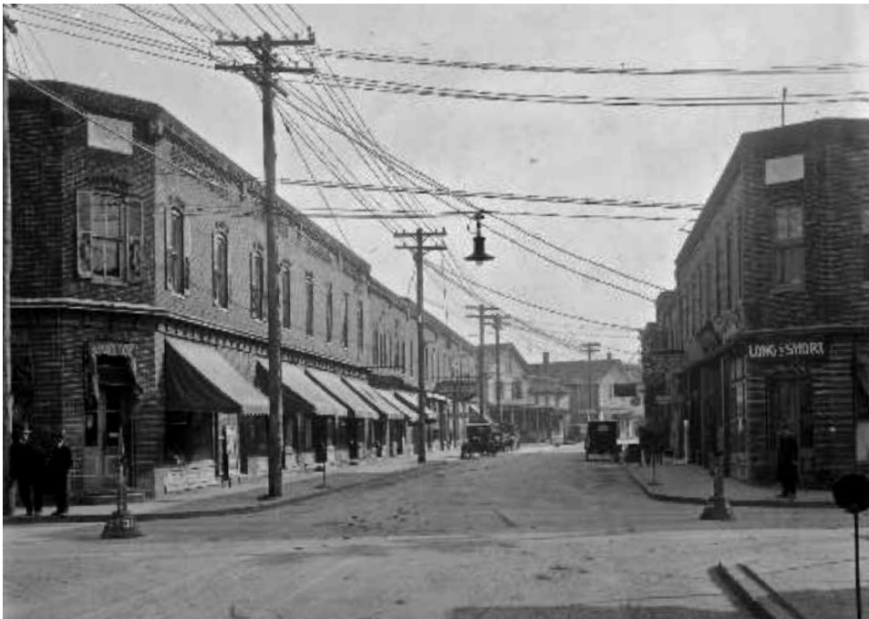
Much of downtown Laurel was made of brick in the 19th and 20th century. These small-scale buildings, most often two or three stories tall, create a pedestrian scale, walkable downtown made for window shopping. Note the many canvas awnings along this street. Source: Laurel Historical Society.
