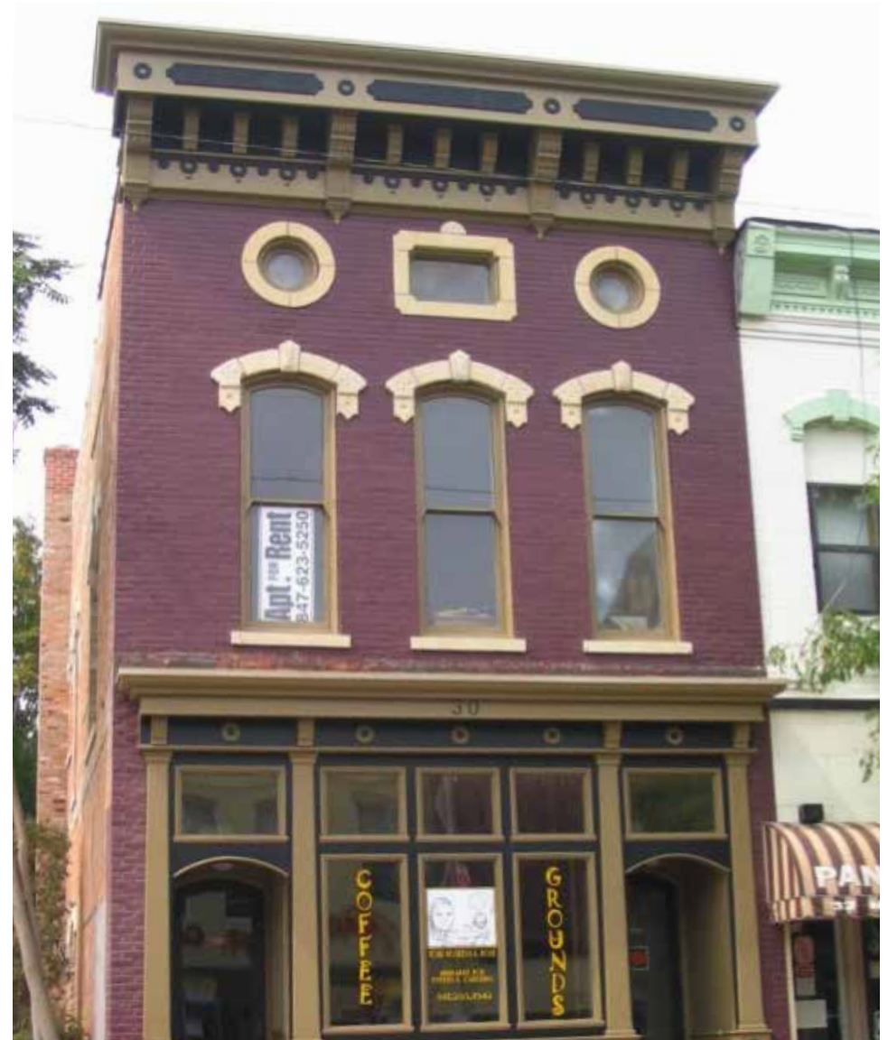
This handsome brick building had been painted several times, but the current three-color combination highlights all of the Victorian historic details on this façade in Geneseo, IL.
