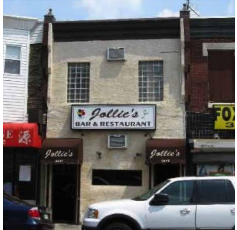
It is not recommended to cover any part of the building façade with aluminum, stucco (seen here), asbestos siding, aluminum siding, simulated brick, surface applied brick and stone, T1-II siding, vinyl siding, Dryvit (exterior insulation finish system), veneer, or any other sheet material. The windows on the second floor of this building in Philadelphia have been infilled with glass block, which is not recommended in Laurel.
