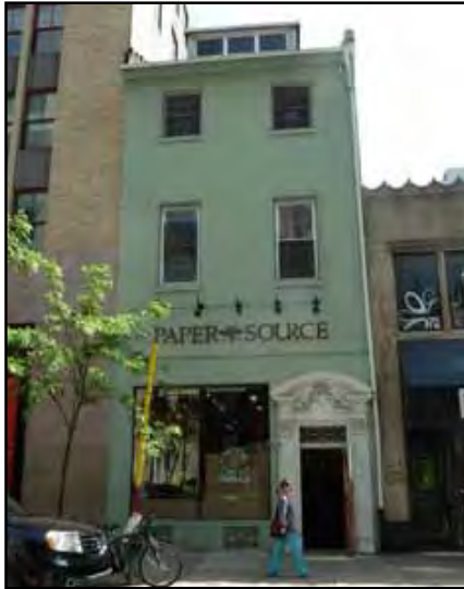
Commercial buildings typically have a long, thin area above the storefront where a sign would be traditionally located.
