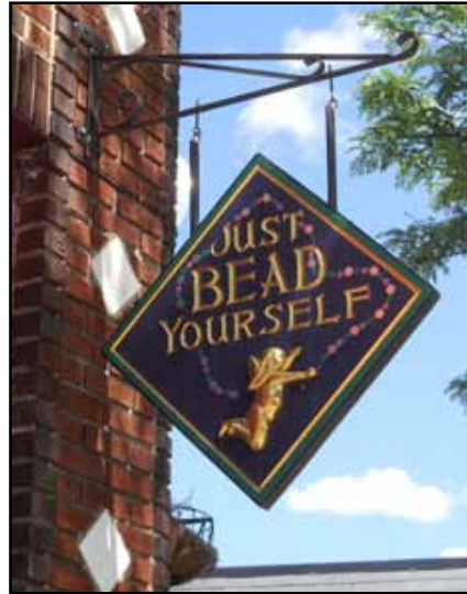
Projecting signs should be placed perpendicular to the building and should have two faces.
