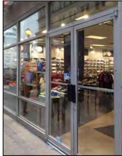
Make sure the interior security grilles and grill box/housing can be completely concealed during regular business hours.
