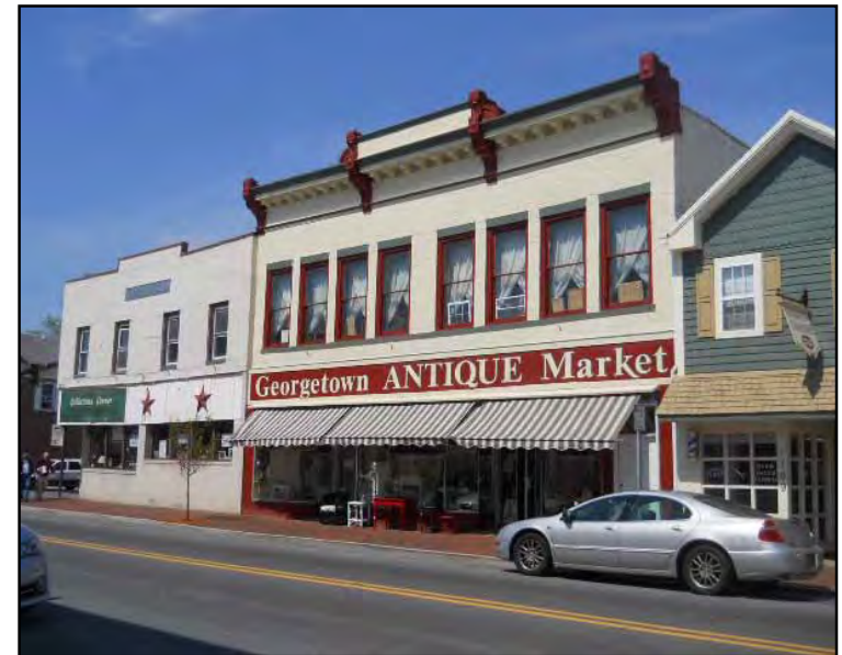
The Georgetown Antique Market is an excellent example of a downtown building that retains its historic appearance, utilizes appropriate colors, signage and awnings, and has been adapted to suit a modern use.
