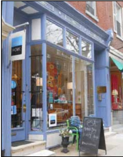
Retain existing large historic storefront windows, their hardware, and framing, as they provide the maximum visibility into the storefront.
