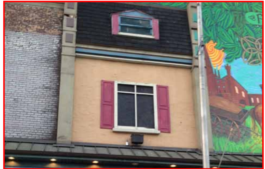
Avoid window shutters unless there is some evidence that they were used historically. .
