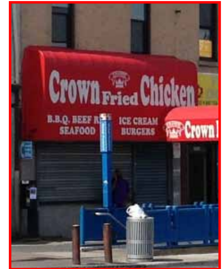
Avoid removing or covering over a historic cornice, whether made of wood or metal.
