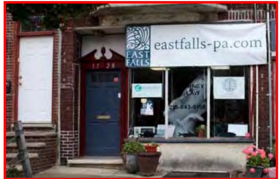
Avoid adding “faux colonial” features or doors that have an abundance of stained or leaded glass.
