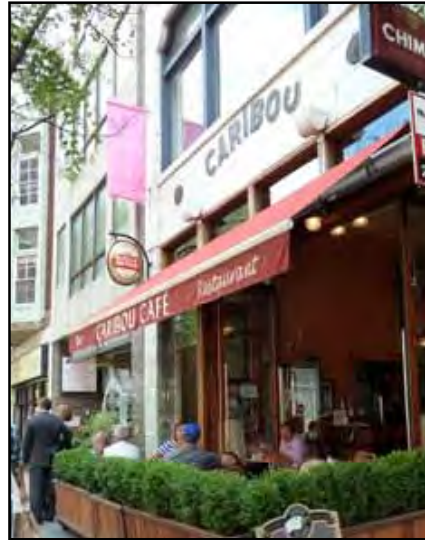
The appropriate zone for signage is generally above the storefront windows and below the sills of the second floor windows.
