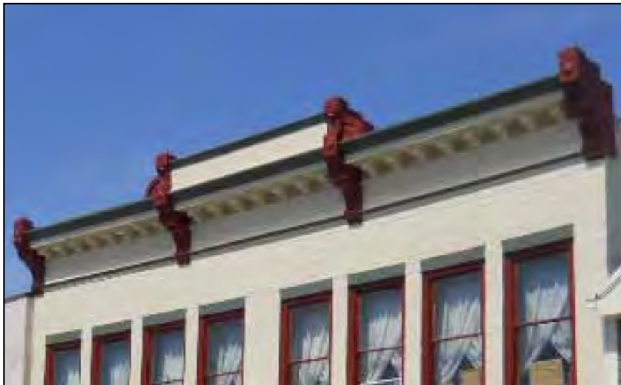
Retain any historic cornice. Keep upper story masonry, wood and metal cornice or parapet treatments intact.
