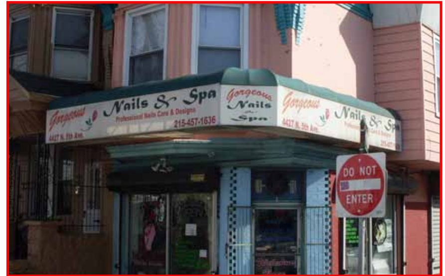
Internally lit awnings, those made of vinyl or plastic, and bubble or rounded awnings on main facades are not recommended.
