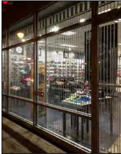
Use open security grilles installed inside the window display glass to allow lighted window displays to be seen at night.
