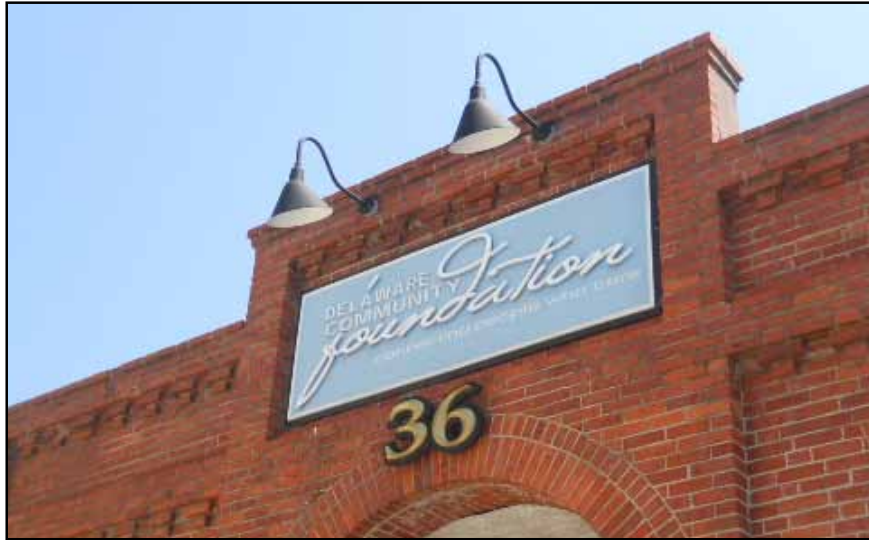
Gooseneck lights provide a good source of indirect lighting for building signage.
