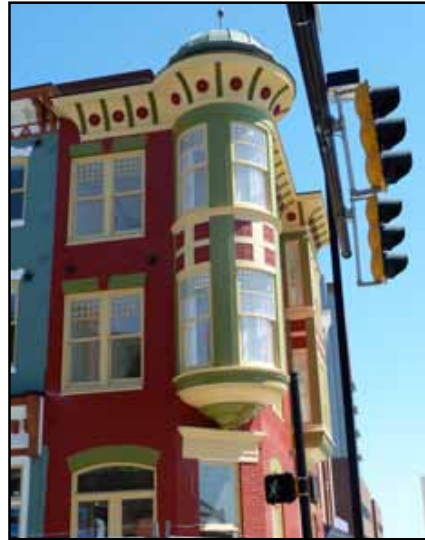
Preserve and restore historical features of the upper facade and cornice.
