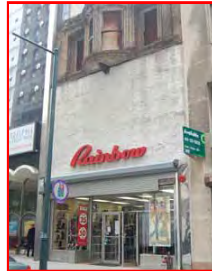
Avoid covering any part of the building facade with aluminum, stucco, false-brick, vinyl siding, veneer, or any other sheet material.
