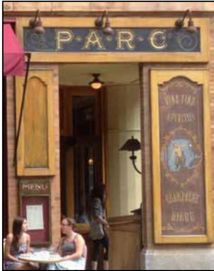
Carefully select typefaces that are harmonious with the building and nature of the business.
