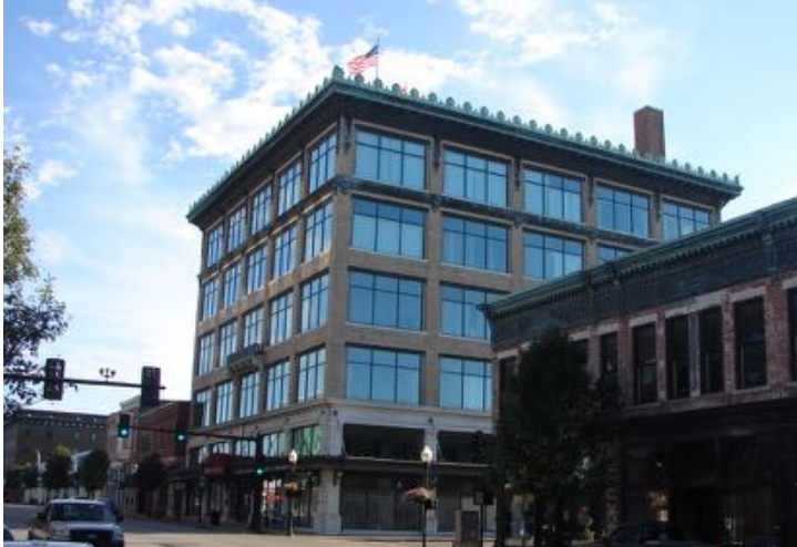
Joplin's five-story City Hall is adapted from an early 20 th century department store.
