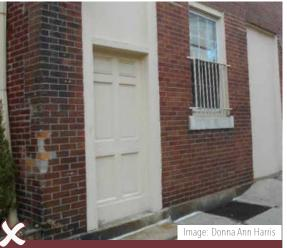
This painted wood paneled door to a residential apartment in Philadelphia has had its transom window removed and replaced with wood. Removing a transom over a door is not recommended in Haddon Heights historic districts. **True Divided Light:** glazed panel in which the glazing is divided into several small panes or "lights" set in the muntins.
