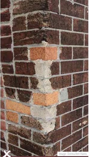
Individual brick units at the corner of this building in Philadelphia have been replaced with brick that does not match the surrounding brick. Several mortar patches have been placed on the corner, rather than brick replacements. The patches and repointing are made with Portland cement, which is much harder than the brick itself. This will cause the adjacent historic brick to spall and eventually disintegrate.
