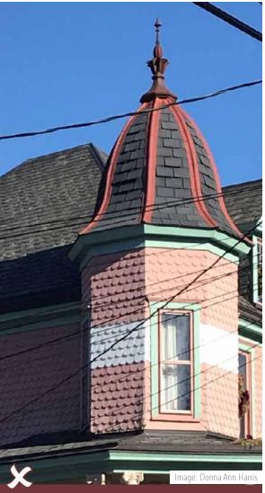
This house in Haddon Township is well restored with a shingle slate roof on the main body and cross gables of the house. However, the roof of the tower has been replaced with asphalt shingles rather than slate to match the main roof. A roof with two different types of roofing materials is not recommended for historic buildings in Haddon Heights.
