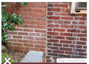
The pointing in the upper left-hand portion of this brick building in Philadelphia has been applied correctly, while the brick pointing on the right side has been poorly applied. The right side shows where the new mortar has been permitted to "feather edge" onto the face of the adjacent bricks, which is not recommended.
