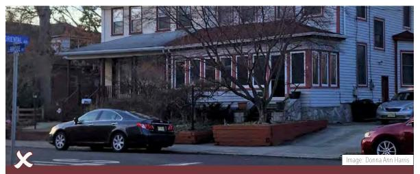
The porch treatments on this twin house in Haddon Township could not be more different. The right side owners have completely enclosed their porch using large single light windows inset into a new wall. The left side owners retained an open porch, but replaced the porch columns with iron posts. It is not recommended to use iron posts rather than porch columns on historic homes in the historic districts in Haddon Heights.
