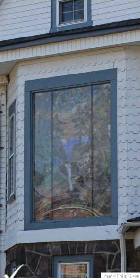
This large fixed stained-glass window at 101 Fourth Avenue is inset into the second-floor bay window. The stained-glass window is covered in plexiglass to protect it. Windows covered in plexiglass should have weep holes in the plexiglass to permit condensation to evaporate.
