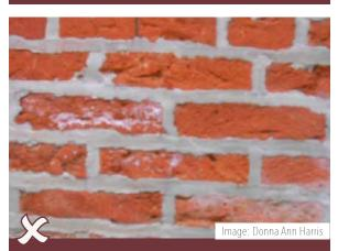
This brick wall was sandblasted at some point in the past, which removed the hard exterior coating on the brick. The brick has also been repointed with Portland cement, which is too hard for historic brick. Sandblasting of brick or stone or use of any other type of abrasive cleaning is not recommended in Haddon Heights.
