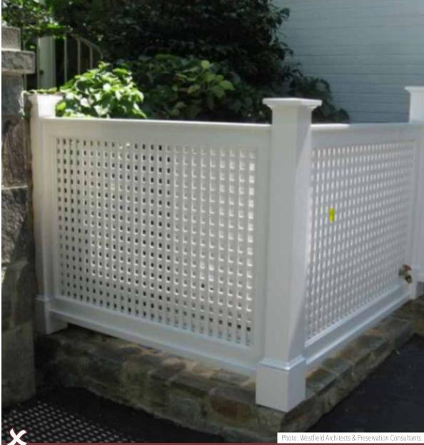
It is not recommended to locate outdoor equipment such as condenser units on the primary or secondary façade of the building. However, if this is unavoidable, it is very important to provide screening such as framed lattice fencing to hide it, as seen here.
