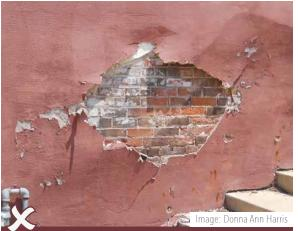
Stucco over this brick wall has been allowed to deteriorate and separate from the wall on a commercial building in Moline, IL. It is not recommended to allow brick, stucco, limestone, or other masonry on historic commercial buildings to deteriorate.
