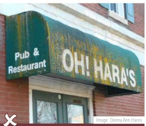
Maintain awnings in good condition. Wash and repair them as needed. This awning from a restaurant in Gloucester City, NJ, needs to be washed or replaced. This awning is also not the proper size or style for the door opening it covers.
