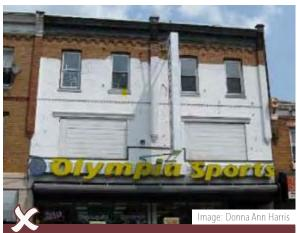
It is not recommended to paint brick (see above), stone, tile, stucco, or molded concrete block if they have never been painted before, as seen on this building in Philadelphia. The unpainted masonry elements have a natural or man-made finish that is important to preserve.
