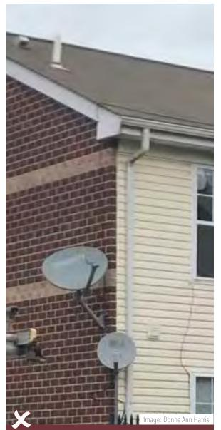
These satellite dishes have been installed on the front façade of this home in Philadelphia. It is not recommended to place satellite dishes on the primary elevation of a building where it can be seen from the public right of way.
