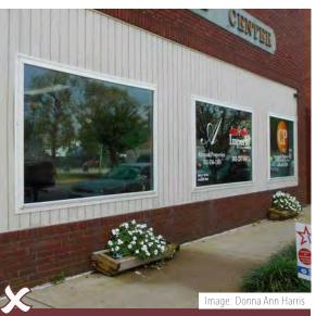
It is not recommended to infill large glass display windows with T1-11 siding or any other solid materials, like this storefront in Seaford, DE.
