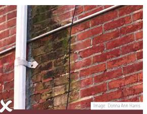
Black stains on this brick wall indicate that mildew is present due to water infiltration, likely from a loose seam on the back of this white metal downspout. Water from the downspout is also washing away the mortar between the bricks. It is not recommended to permit downspouts to leak and cause damage to the adjacent brick in Haddon Heights.
