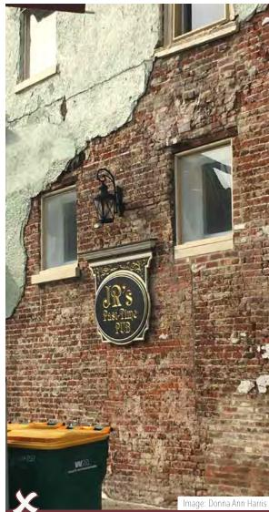
On a rear façade of a commercial storefront in Smyrna, DE, this owner has allowed the stucco to delaminate (come away) from the brick. The brick underneath the stucco has not been repointed, making the wall vulnerable to further deterioration from water infiltration from rising damp or rain.
