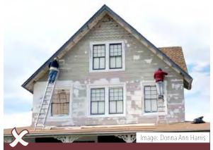
It is not recommended to permit historic buildings clad in wood (either clapboard or shingles) to deteriorate due to lack of paint in Haddon Heights. This house in Beach Haven, NJ, is being scraped and primed before painting to assure a quality paint job. A good paint job with proper preparation can last between 8 and 10 years.
