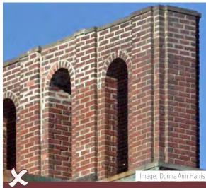
It is not recommended to use hard Portland cement-based mortar on historic masonry constructed prior to 1930, as seen on the top portion of this historic chimney.
