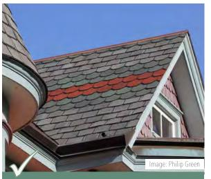
Retain any decorative slate roof, such as the one found here at 107 Fourth Avenue. This roof uses an elaborate three-color scheme of gray, dark green, and red colored roof shingles. Note the copper gutters and downspouts.
