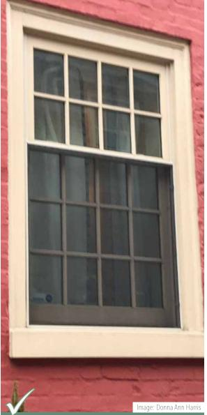
Double planed, vinyl clad wood windows with true divided lights can be made to fit most window openings, like this eight over twelve light sash in Philadelphia. This one has a movable bottom screen.
